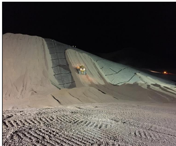
Night time ODF placement
